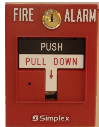
Figure 5 Typical Fire Alarm Pull-Station
