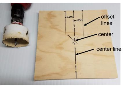
**Step 2:** Drill a 3" diameter hole in the center of the part with a 3" diameter hole saw.
