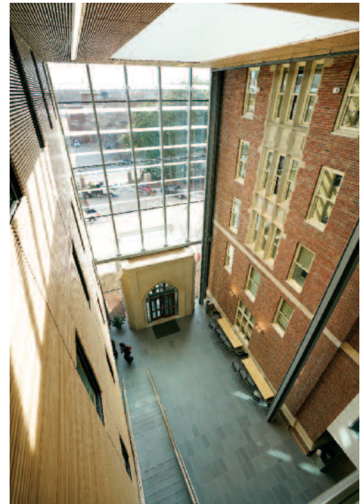
▲ Above: The existing exterior wall of historic Godchaux Hall forms one side of the atrium. Opposite: The monumental staircase is self-supporting with no visible support beams that block light.
