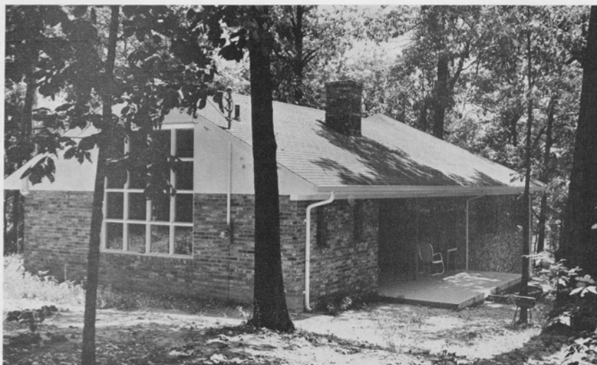
The director's residence on the grounds of the Dyer Observatory.
