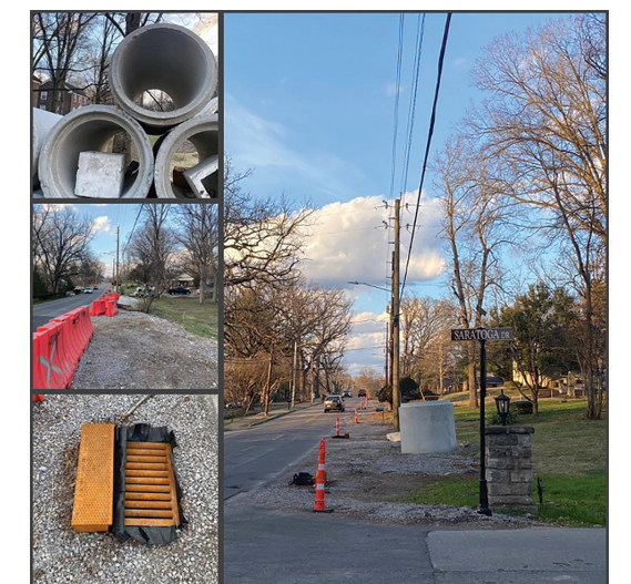
Case study of current sidewalk construction project underway on Bowling Ave near Saratoga Dr. In this case, using conventional stormwater management practices necessitates the installation of curbside inlets and pipes of up to 39" beneath the right of way.
