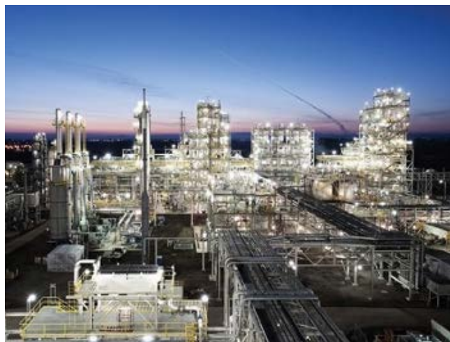
The REC Silicon plant in Montana uses the Union Carbide Process, with alternating reactors and separators to manufacture silane, while using recycle streams to minimize waste.
