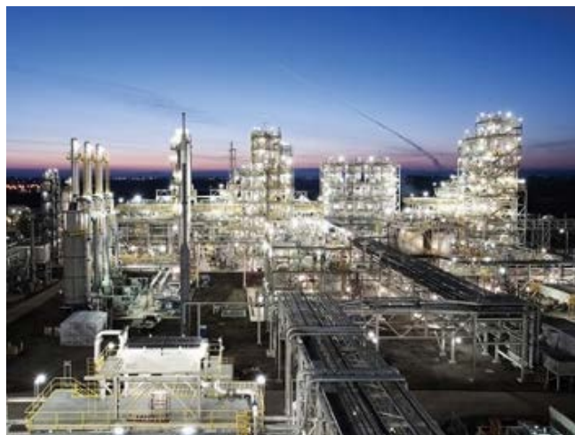
The REC Silicon plant in Montana uses the Union Carbide Process, with alternating reactors and separators to manufacture silane, while using recycle streams to minimize waste.
