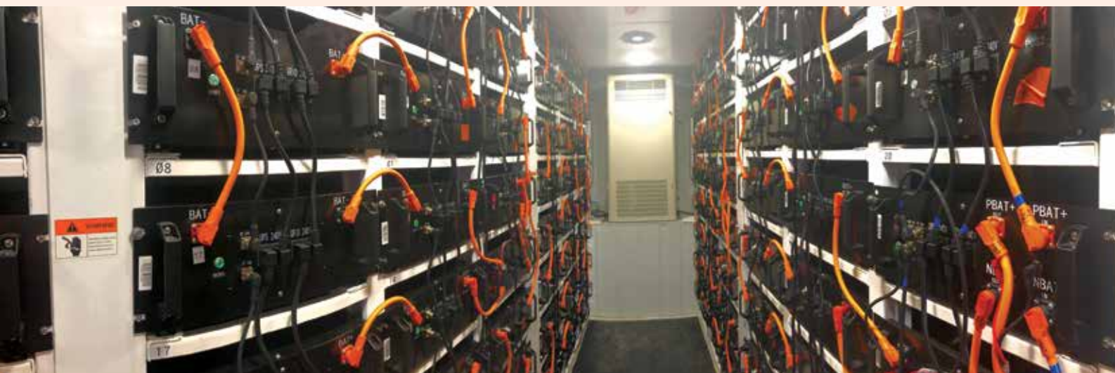
Gridspan's modular battery assembly is housed in an air-conditioned shipping container. The container is easy to relocate and can be shipped, trucked or transported by train.
