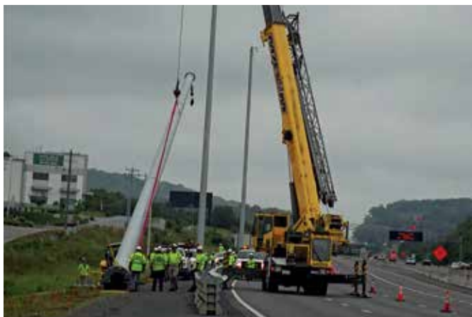
High-resolution cameras atop poles along the I-24 corridor will provide real-time vehicle trajectory information using computer vision algorithms.
