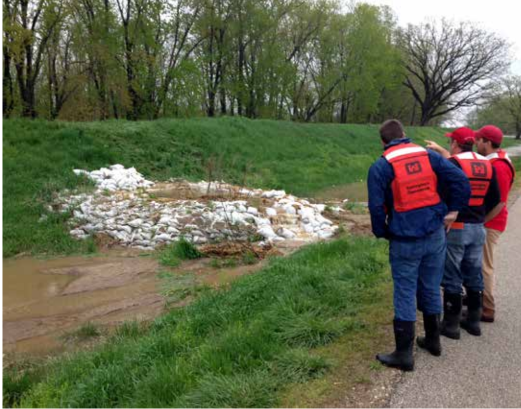
Above, The Army Corps of Engineers works to control seepage and resulting sand boils under the Mississippi River mainline levee near Memphis, Tennessee, in February 2019. Photo: Army Corps of Engineers, Memphis Division.
