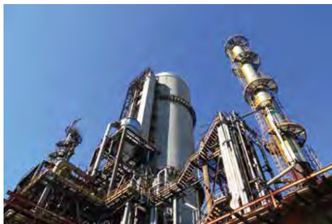
A typical sulfuric acid plant
