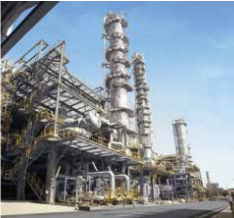
Distillation columns are common in chemical plants and they require a lot of utilities. Heat and mass integration could heavily reduce their utility consumption.
