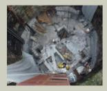
Step 3: Dig a huge hole. To do this, you must first dig small holes with rock drills, then use explosives to blast the rock. Dig more small holes, blast more rock, dig, blast, and so on until you have achieved your large hole, 100 feet deep with a diameter of 60 feet. This may take awhile.
