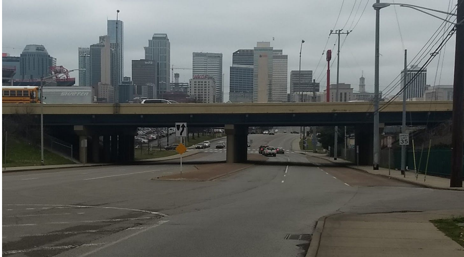
Figure 3. Woodland Street Underpass
