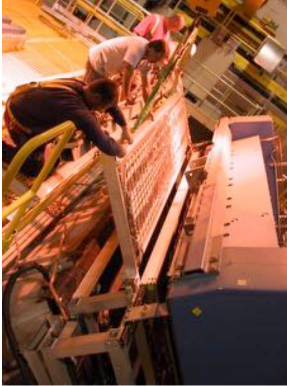
FIGURE A.5. Top of Central Arm West, in the process of installing one TOFW sector
