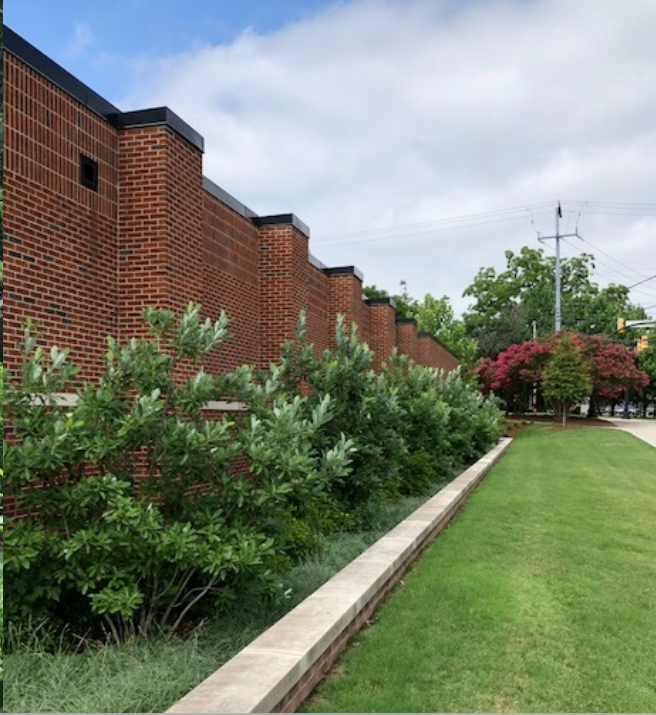
McGugin Bioretention Area
