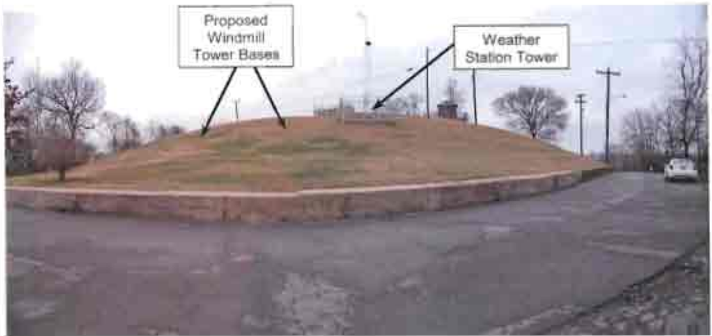
Photo 1: The Love Circle site is shown in this panorama photograph. The arrows point to the approximate locations for the planned windmill towers. An underground water reservoir is located inside the hilltop. The construction of the approximately 20 ft deep reservoir was apparently about half into the hill and about half behind a wedge of fill.
