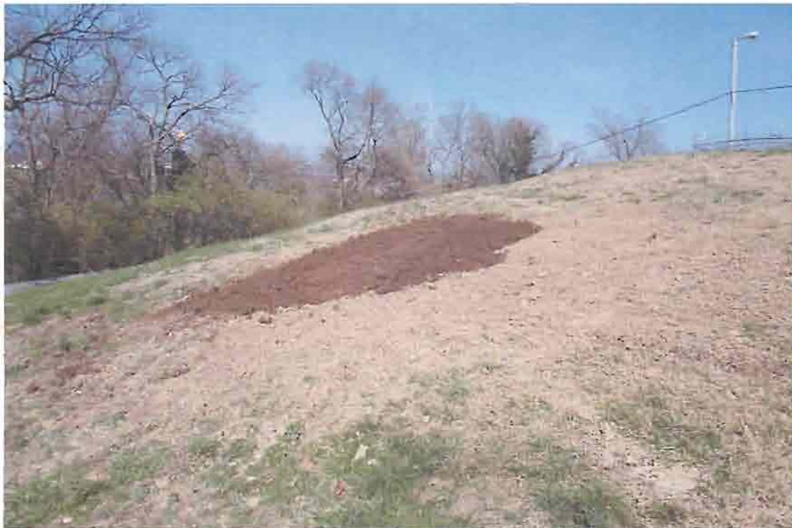
Photo 4: The Test-Pit TP-1 was finished off with about 5 yd 3 of topsoil brought in from off site.
