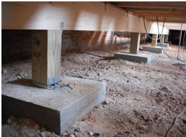
Figure 2: Pier and Beam Foundation<sup>5</sup>
