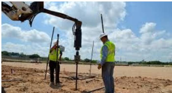
Figure 8: Helical piers screwed into the ground provide cost saving benefits<sup>43</sup>
